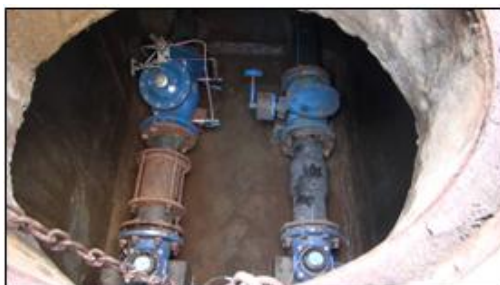
Figure 3. Installation of Smart Water Meter
