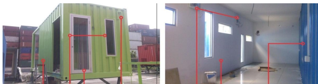
Figure 5 - 6. Installation of pipeline utility and fittings (Courtesy: Magnus Cipta Estetika, Pte.Co)
