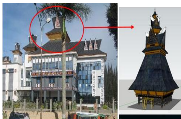
Figure 5: The View of Karo Regency Office Building Roof
