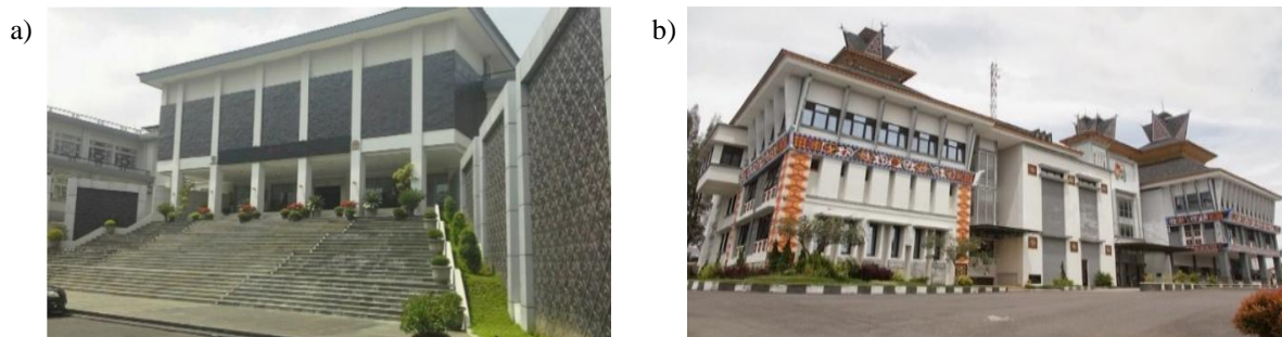
Figure 3: DPRD Bandung Building (a) and Karo Regency Office Building (b)
