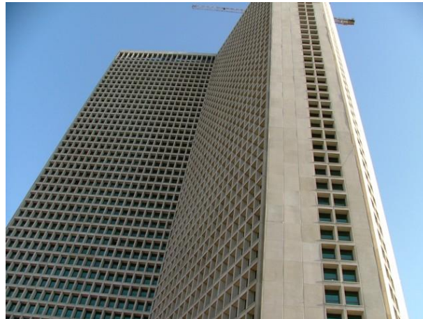
FIG.16. material and windows in Tehran tower
