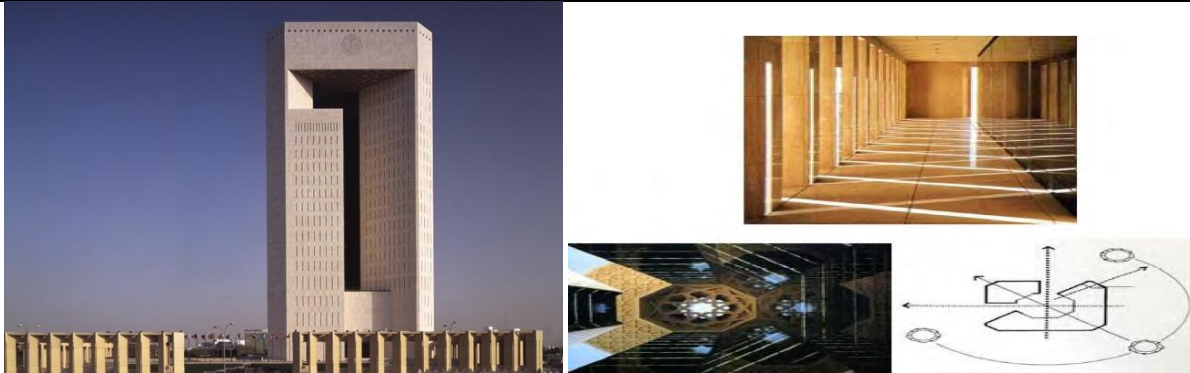
FIG.11 & 12. Islamic Development Bank, Jeddah. Nikken Sekkei Architects
