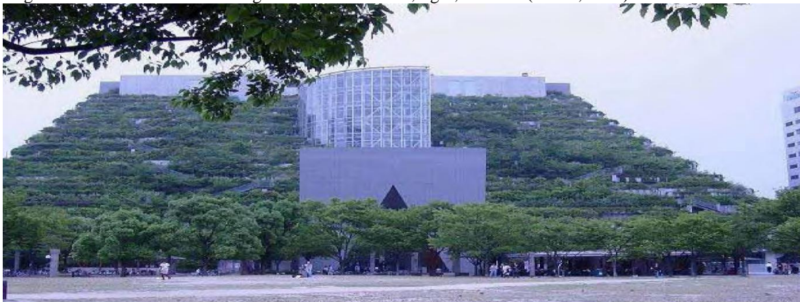
FIG.2. ACROS Fukuoka Prefectural International Hall, Japan. Emilio Ambasz and Associates.1994
