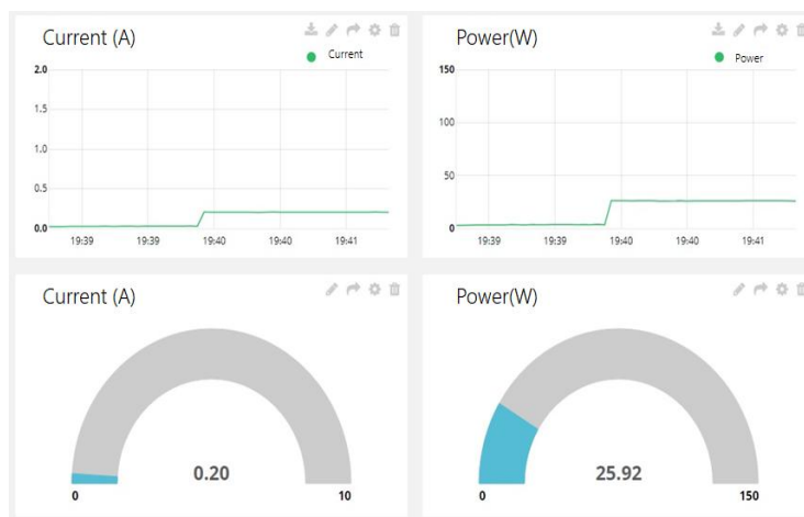
Figure 11: Monitoring of electrical current and power
