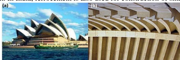
Figure 1: Sydney Opera House (a) Front view (b) Shell ribs
