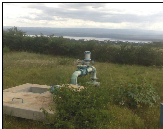
Figure4: NAWASSCO borehole outlet at Naka area, with Lake Nakuru in the background.
