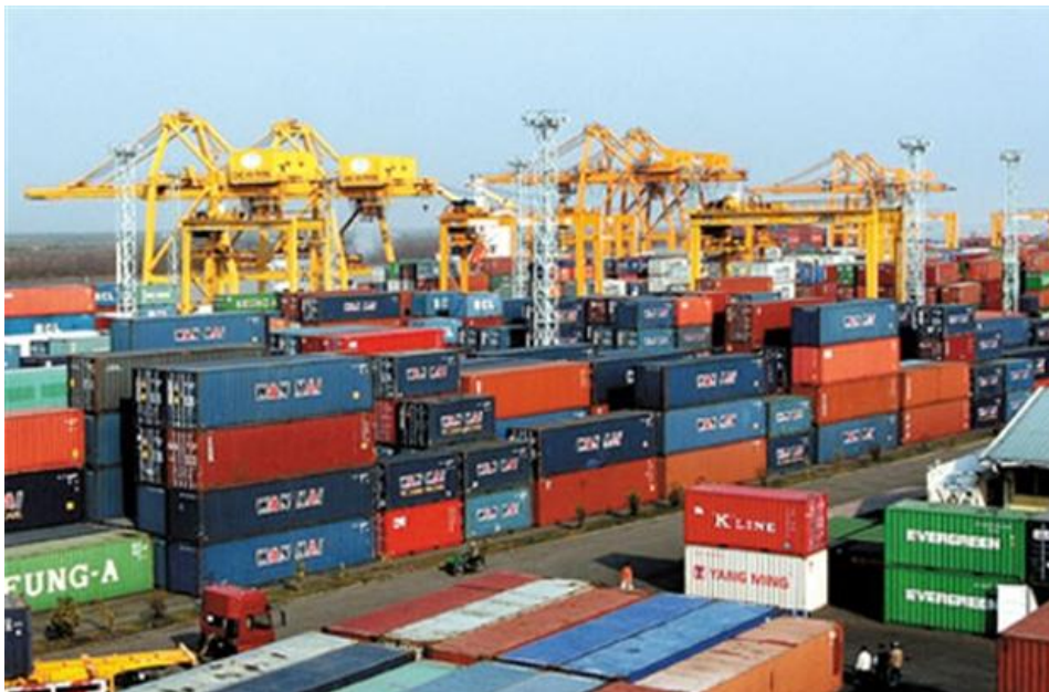
Figure 1. Service seaport in a port, Vietnam
