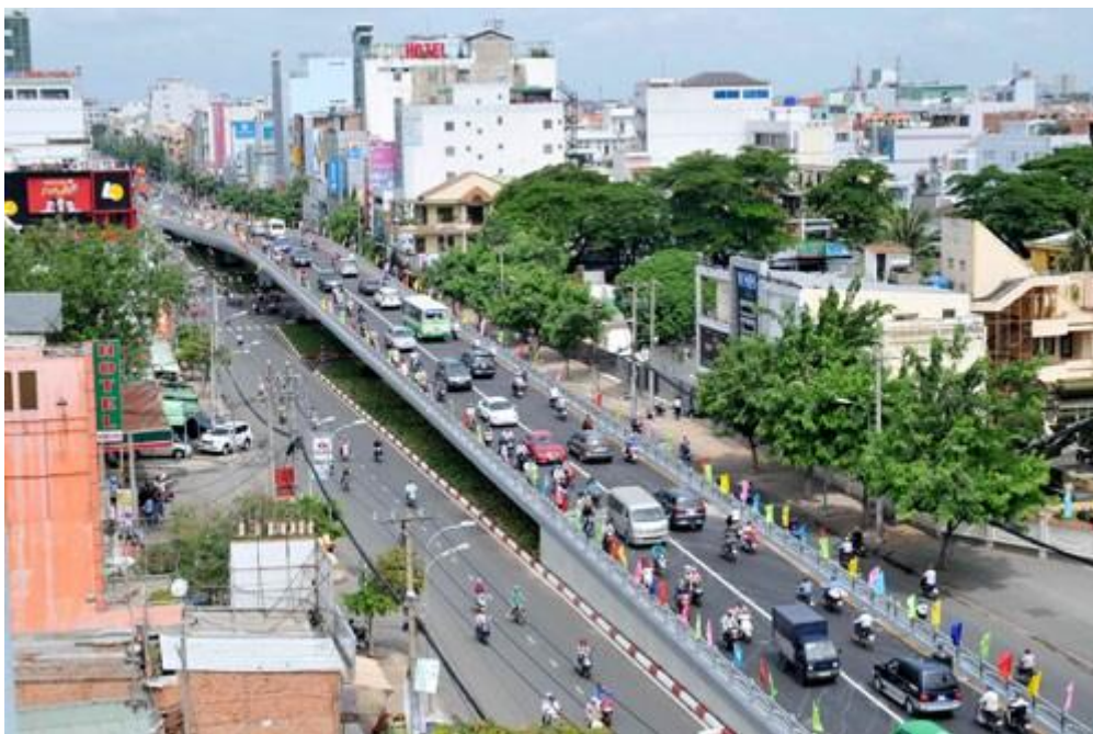
Figure 1. Overpass bridge to reduce the traffic jam
