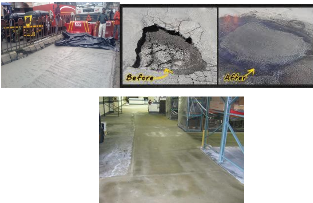
Fig 2.6 shows the ACC supercoat used to fill the potholes in roads
