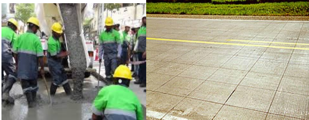
Fig 2.5 Shows the ACC speedcrete concreting work
