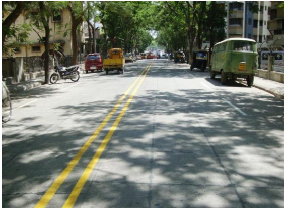
Fig 3.1 shows the paper cutting and road done with UTWT -24
